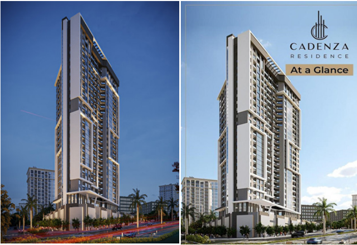
Figure 2- CADENZA RESIDENCE, 1 Katonga Rd, Kampala-24 floors at a height of 80m
