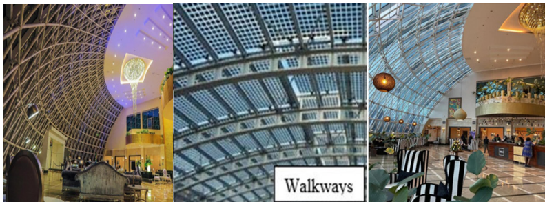
Figure25- Double-glazed BIPV window with ventilation before and after installation on walkways
