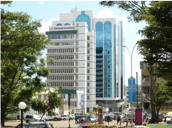
Figure 4- Workers' House- 20 Floors at a Height of 72.33m
